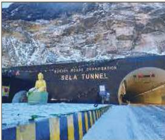
Sela Tunnel Delivered March 2024
