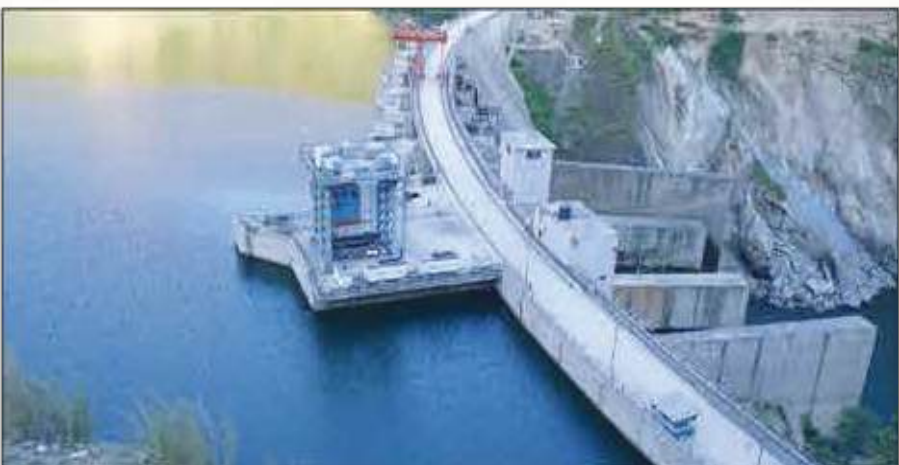
Kameng Hydro Electric Project Delivered November 2022
