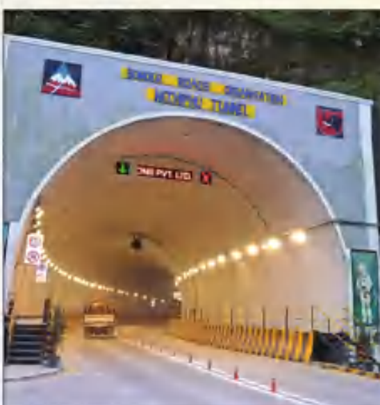
Nechiphu Tunnel Delivered September 2023
