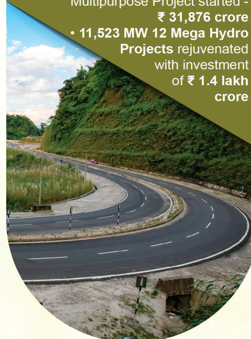
₹ 44,000 Cr for new 2,574 km National Highways
